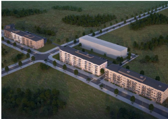
Fullerö 21:73 Uppsala SEK 143mn Sweden Green Building Council (Silver)
